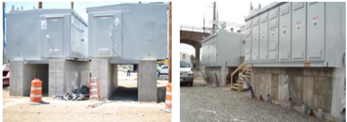
Figure 6. Far Rockaway (left) and Arvene (right) substations after implementation of storm hardening projects.
