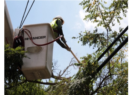
Figure 3. A tree trimming crew maintaining
