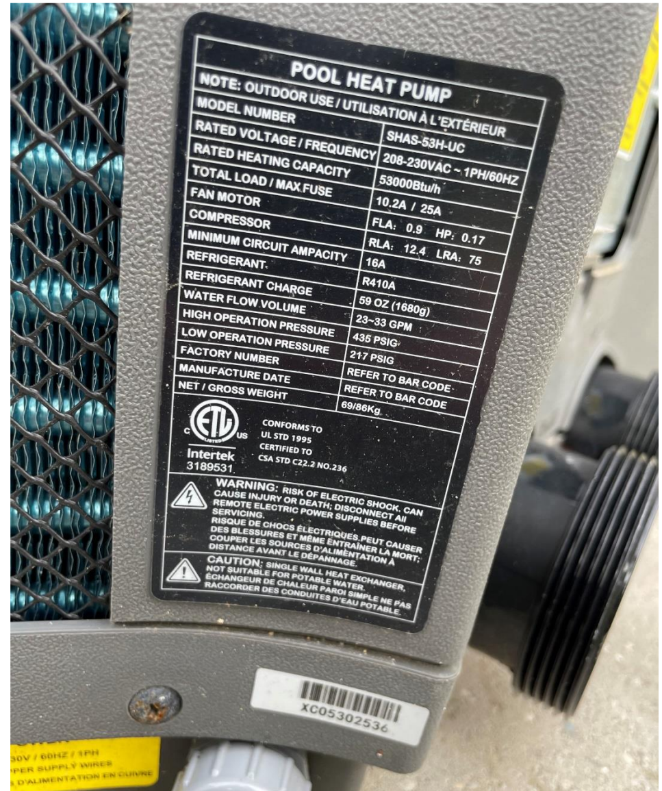
Example of Installed Heat Pump Model Number/ Serial Number Tag on the Unit
