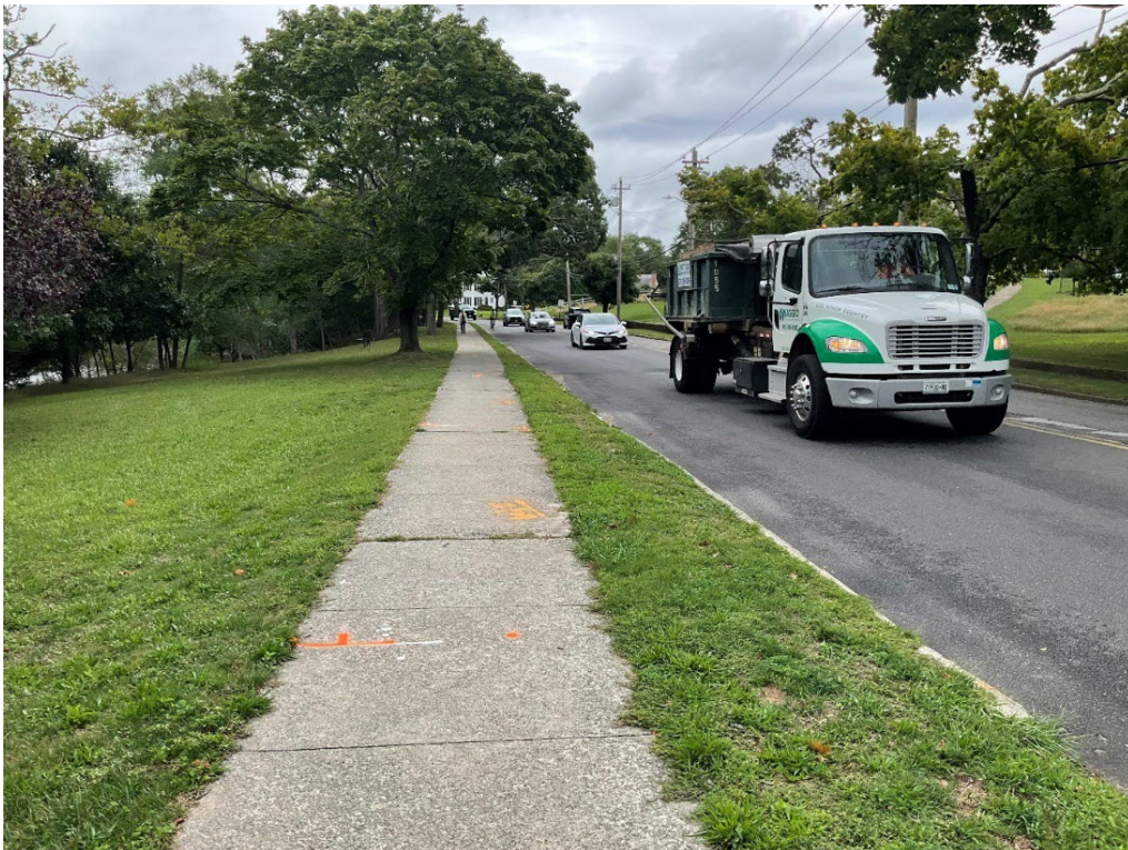
Photograph A-6. Utilities and sidewalk along Jermain Avenue in the Village of Sag Harbor precluded the area from testing in this survey (Chronicle Heritage, August 2024).
