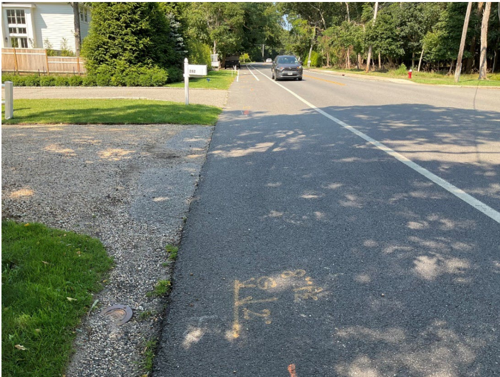
Photograph A-8. Gas main cap in gravel (left foreground) indicates buried utilities on Hampton Street (Route 114). Opposite side of the street tested in this survey (Chronicle Heritage, August 2024).
