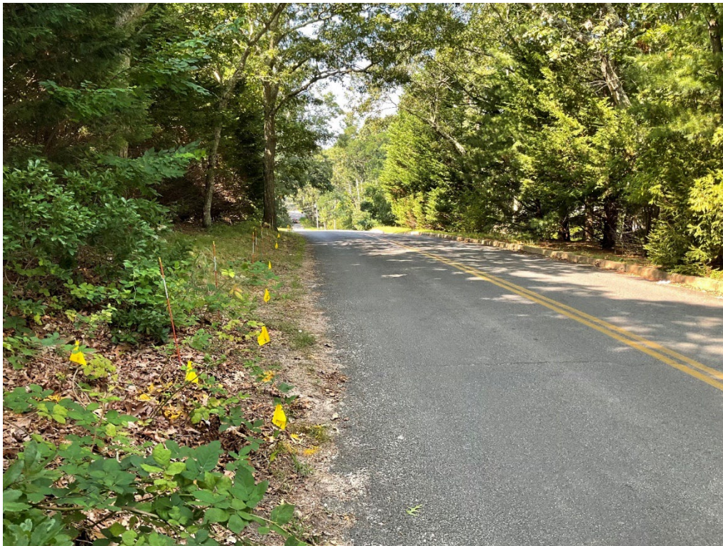
Photograph A-16. Gas main mark-out (yellow flags) on southern side of Harrison Street. Reflector poles mark the edge of the ROW and narrowness in some areas (Chronicle Heritage, August 2024).
