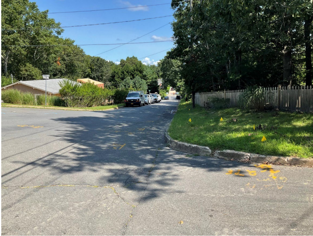
Photograph A-17. View showing gas main on eastern side of Harrison Street Extension showing narrowness of ROW (Chronicle Heritage, August 2024).
