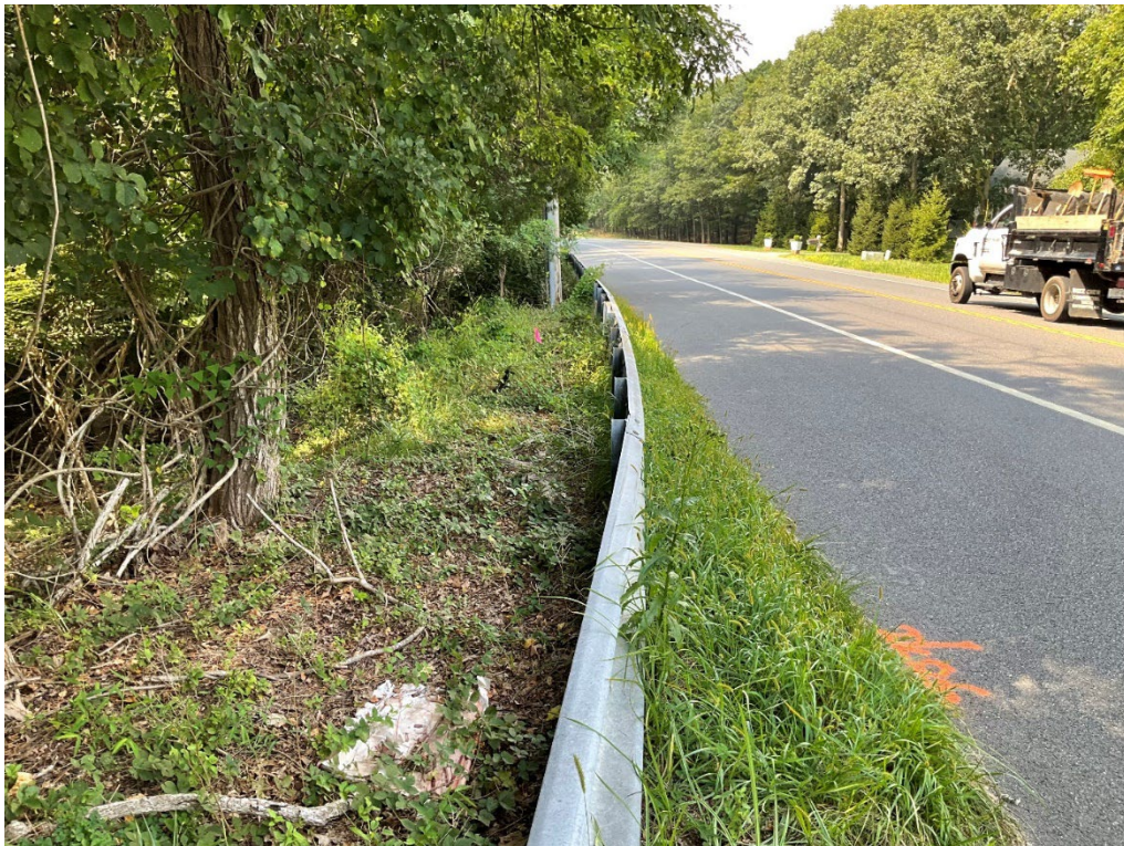
Photograph A-14. Small testable area on southern side of guardrail, southern side of Route 114. Utility pole and sloping ground surface in middle ground (Chronicle Heritage, August 2024).
